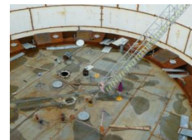
BP Tank Refurbishment
