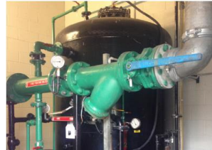
AFFF storage tank recertification at RAAF Townsville for JLL
